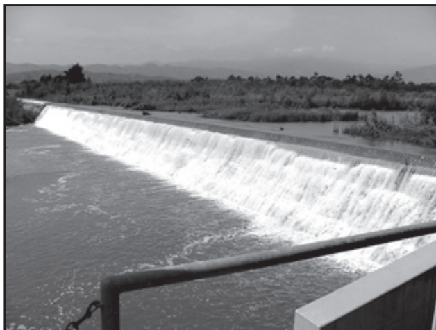
Winter storm flows passing over the Freeman Diversion Dam on the Santa Clara River near Saticoy.
